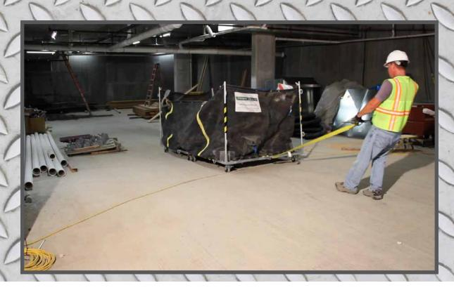
The Surface Dolly can be moved by hand or attach the tow bar and it can be towed with a forklift or other equipment.
