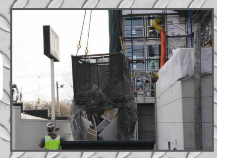
Once Cranetainers are filled, they can be emptied into a large receptacle (e.g., dumpster or dump truck) for materials to be hauled away.
