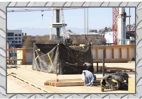
Cranetainers are collapsible, set up quickly, and roll up for easy storage. Because of their small footprint (L-9 ft/W-5 ft/H-4 ft) and light weight (empty weight, 80 lbs.), multiple Cranetainers can be set up where needed to enable continuous production.
