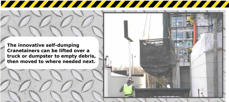
Once the Cranetainer is positioned, the release mechanism is pulled and material safely flows into the receptacle.
