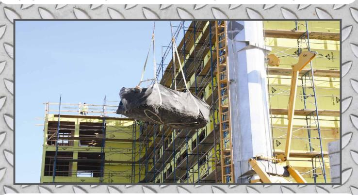
Labor costs are further reduced because the Cranetainers offer greater portability. Once Cranetainers are filled, they are easily lowered to the ground where they can be positioned for emptying, or stored until a receptacle arrives on-site.
