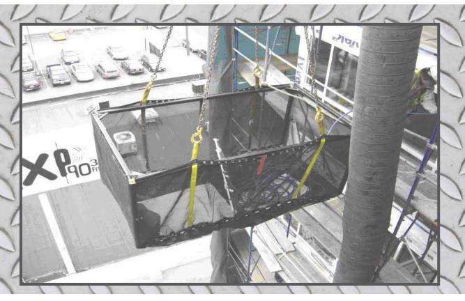
The Aerial Frame allows the Cranetainer to abut any opening where debris can be loaded, such as scaffolding, windows, or sliding doors.
