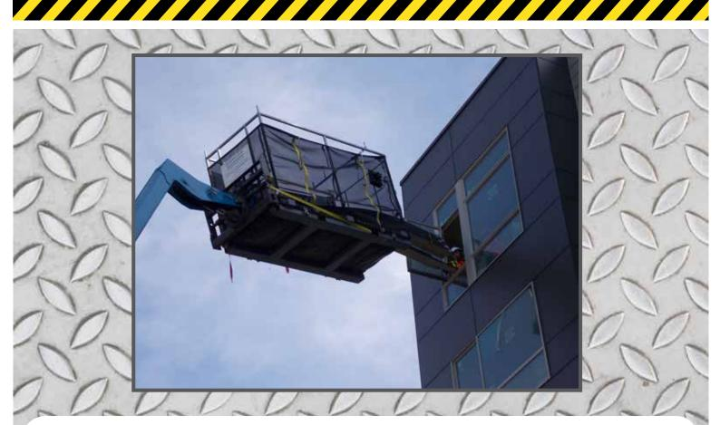
By loading long materials using the Vertical Stabilizer and Stabilizer Extension, workers can place materials through a sliding glass door opening or near a window opening for offloading. Material Handlers can be operated using a crane or, with the addition of a Cranetainer System Forklift Rack, they can also be operated using a forklift.
