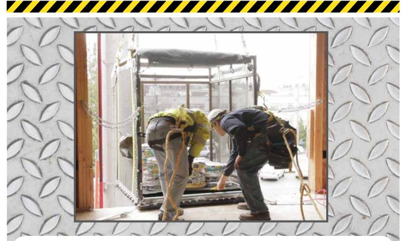
Once positioned in the building opening, the Material Handler is chained off, the cover removed and the material is pulled safely into the building. Unlike conventional wooden boxes and offload procedures the high strength Roller Table requires minimal physical effort to move materials into the building.
