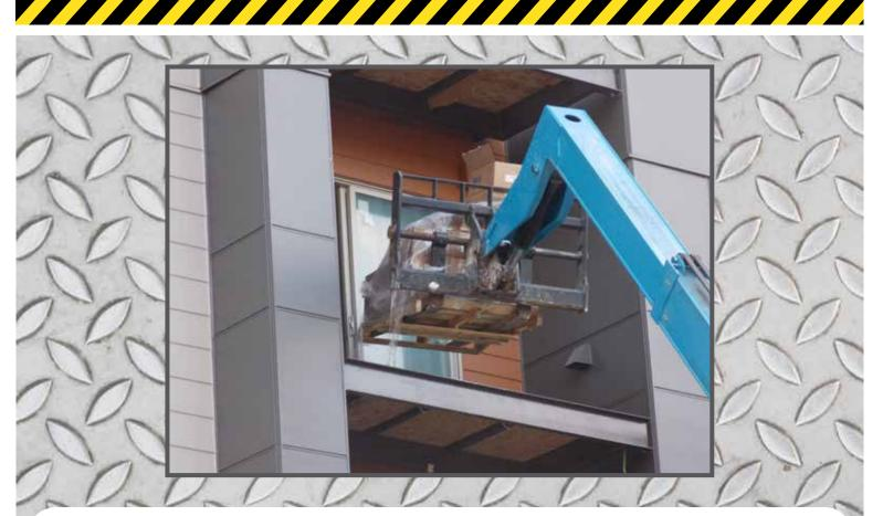
Conventional practices of lifting open pallets and non-secured loads can contribute to workplace injuries due to hazardous offload procedures. Also, non-secured loads increase exposure to property loss due to material damage or falling objects. Material Handlers secure all materials and prevent objects from falling while they are positioned overhead.
