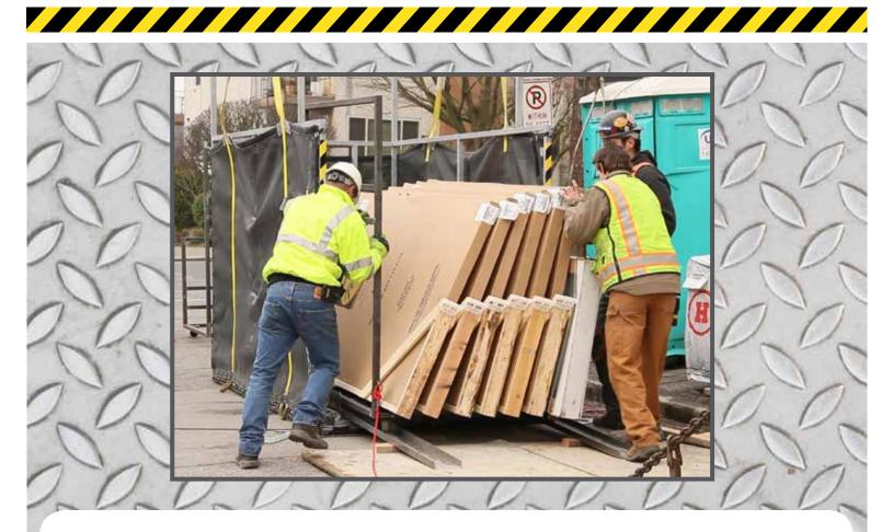
As materials are loaded onto a Material Rack in the loading area below, the other Material Rack is being offloaded into the building above. This continuous workflow dramatically decreases the amount of time it takes workers to load and unload materials.
