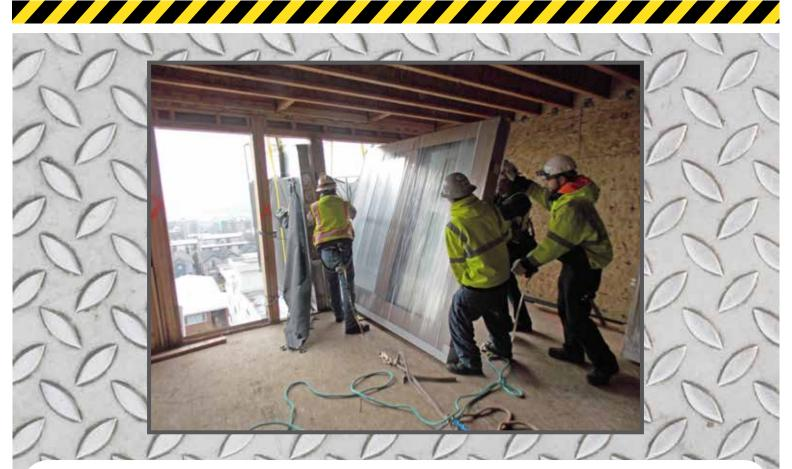
The two different sized Material Handlers allow workers to move any object, including this 430 lb., 8' tall sliding glass door, with much greater ease than conventional wooden boxes. The adjustable Base Stabilizer allows the back of the Material Handler to rest safely for proper loading from trucks with shorter tailgates.
