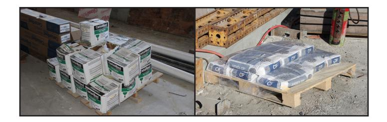
Flying pallets with slings can be hazardous because the pallet slats can break causing loads to shift and possibly spill. Also, materials are often not wrapped or secured safely to pallets and sometimes materials come non-palletized.
