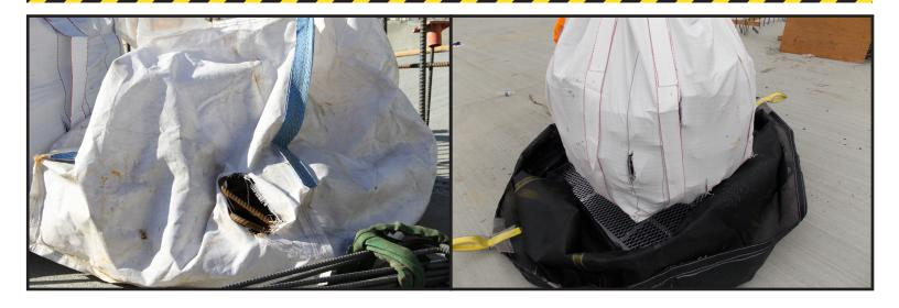
FIBC sacks and one time lift bags can often have tears or holes in them which can cause a hazardous, non-compliant lift. These lifts can be placed into the Quick Hoist and then safely moved around the jobsite.
