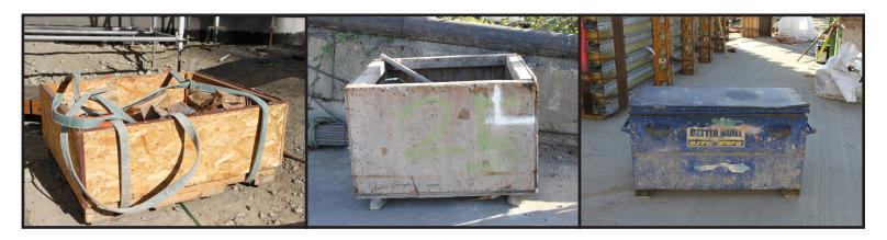
Sometimes homemade boxes and other contraptions are not load rated or certified for lifting. These can also be placed into the Quick Hoist and safely moved around the jobsite.
